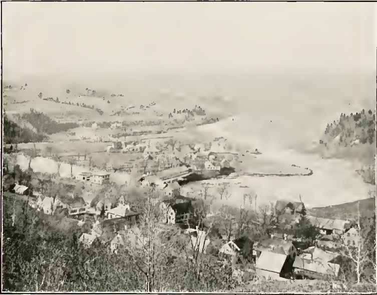
VIEW OF RIVER STREET FROM THE EAST HILL.
