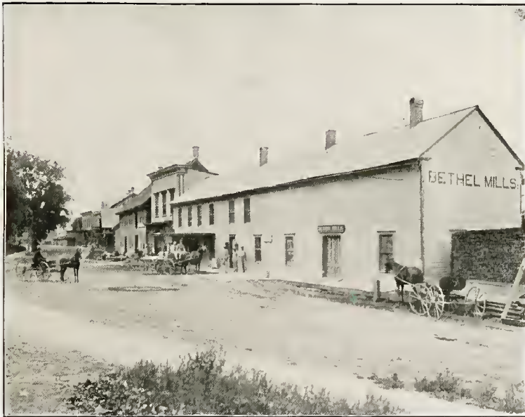
WEST SIDE OF MAIN STREET AND WRIGHT & CUSHING MILL.
