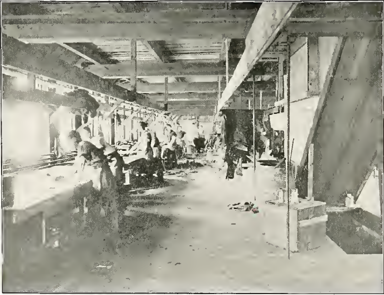
A PART OF EAST SIDE OF FINISHING ROOM.
